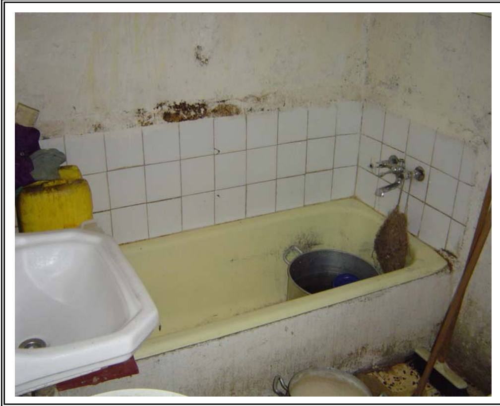
Pictures 3 & 4: The previous bath room
